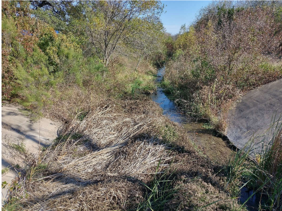
Susan Channel East – Vegetation growing in the channel bed east of Block House Drive
